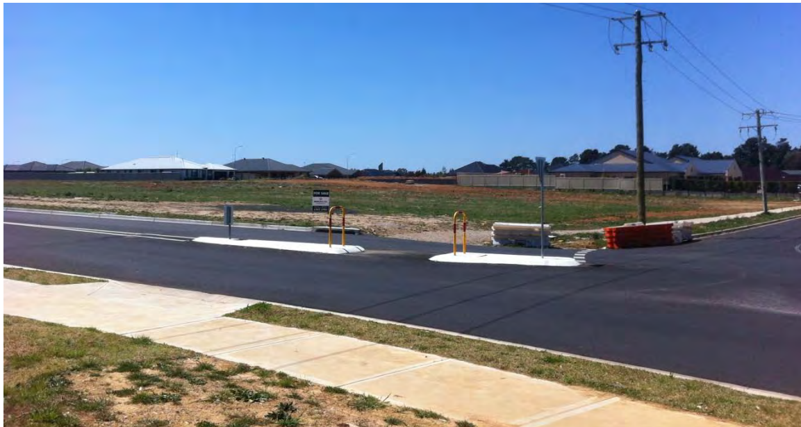
Photograph 1: Site as viewed from the corner of Telopea Way and Farrell Road
